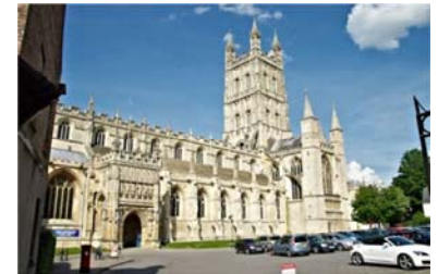
Front view of Gloucester Cathedral. Above the South Porch (left) was a set of six saints statues. Photographed: 19/05/2014
